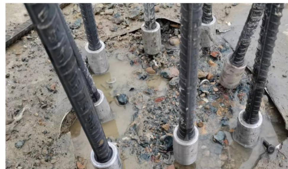
灌注桩钢筋的连接Connection of filled steel bars
