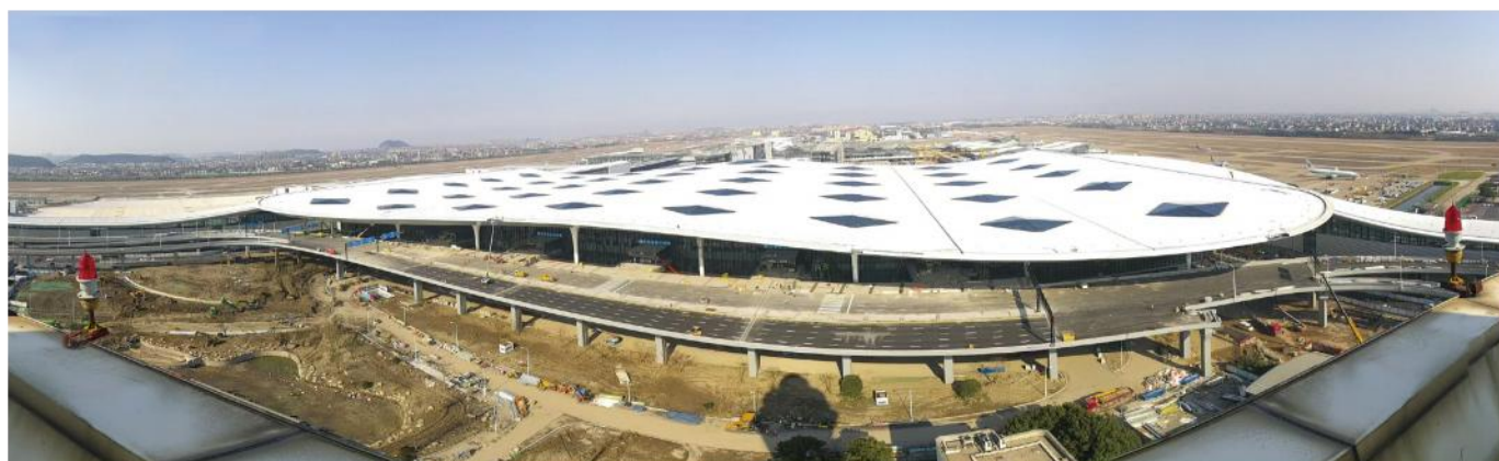
杭州萧山机场扩建 Hangzhou Xiaoshan Airport Project
