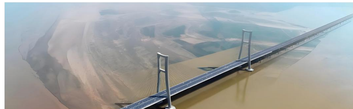
安罗黄河高速 Anluo Yellow River Expressway Project
