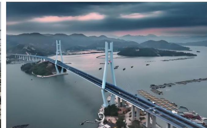
福鼎沙埕湾大桥 Shachengwan Bridge Project
